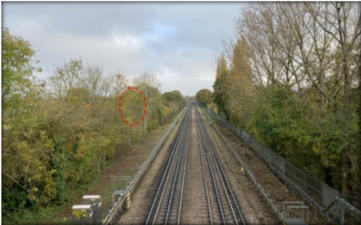
Figure 1: Annotated photograph highlighting the location of T1 – Oak in the landscape, as viewed from the railway bridge.
